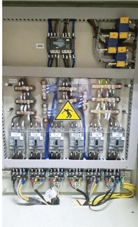
Gambar 4.4 Panel Proteksi Sumber: Zainul/Kemendikdasmen (2024)
